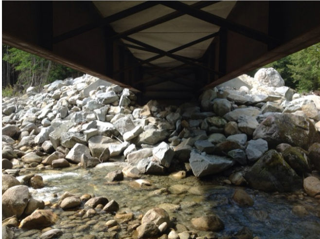
Left Bank Abutment when facing downstream
