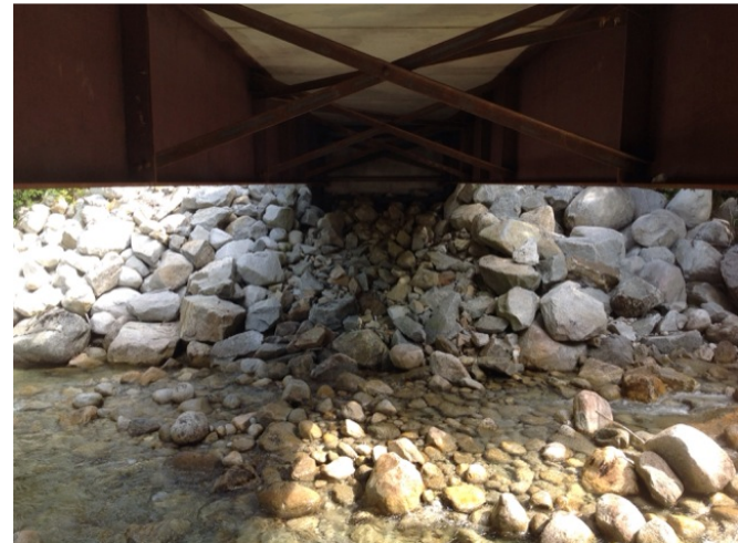
Right Bank Abutment when facing downstream
